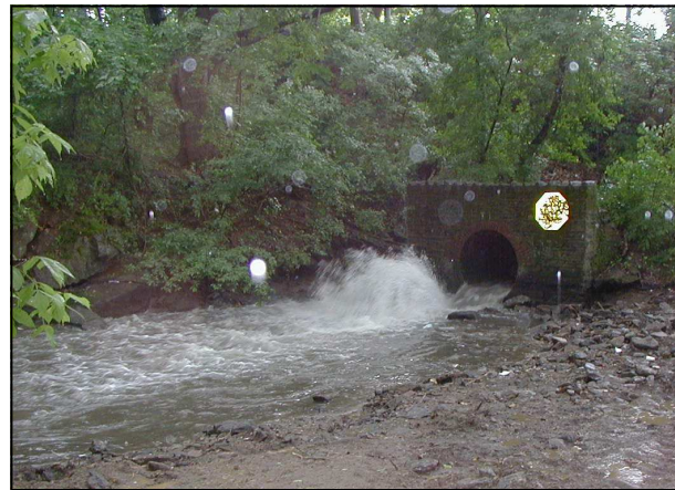
Combined Sewer Overflow at Crescentville in Philadelphia
